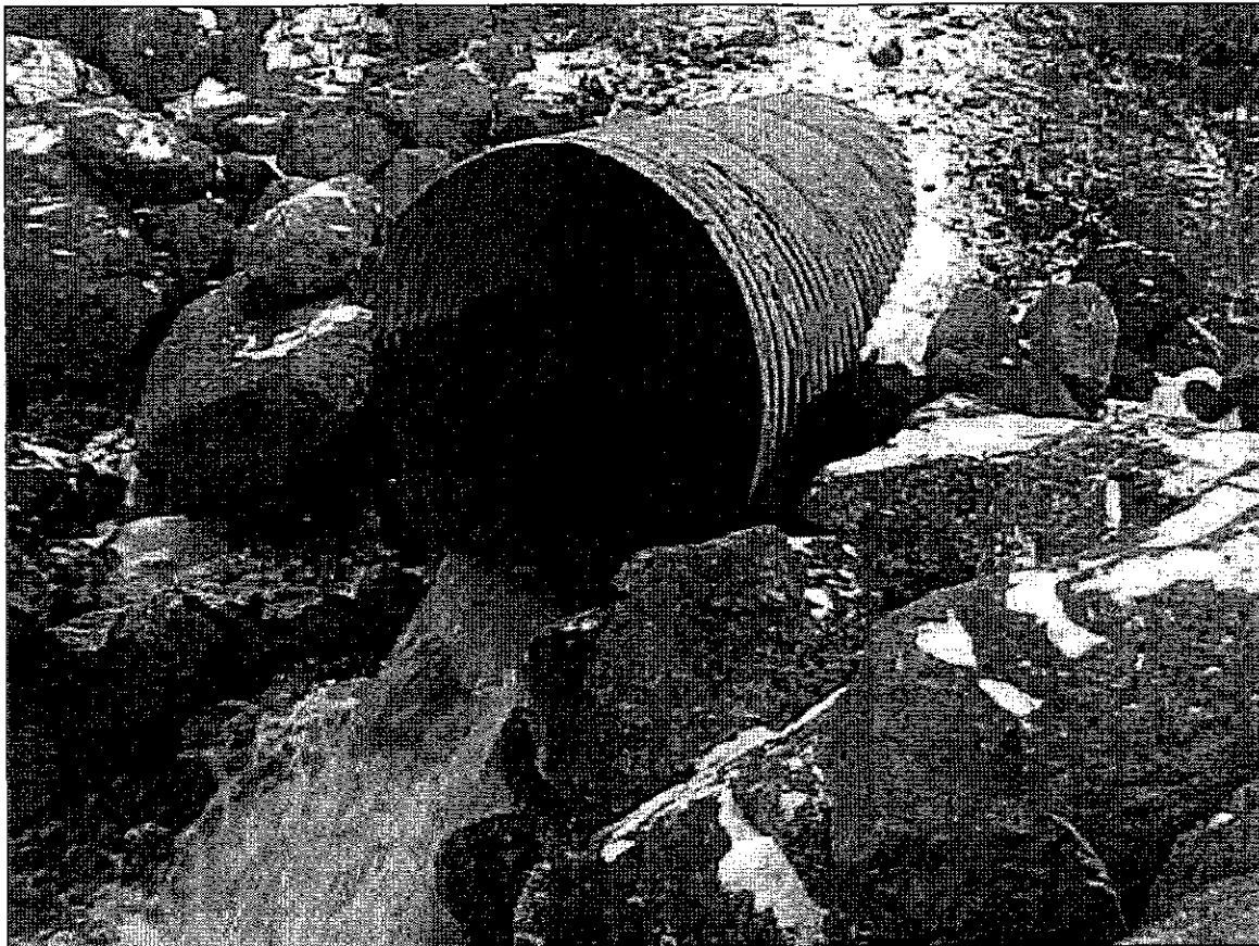
Fenelons Pond Outlet Culvert – Leaking with Gate Closed
