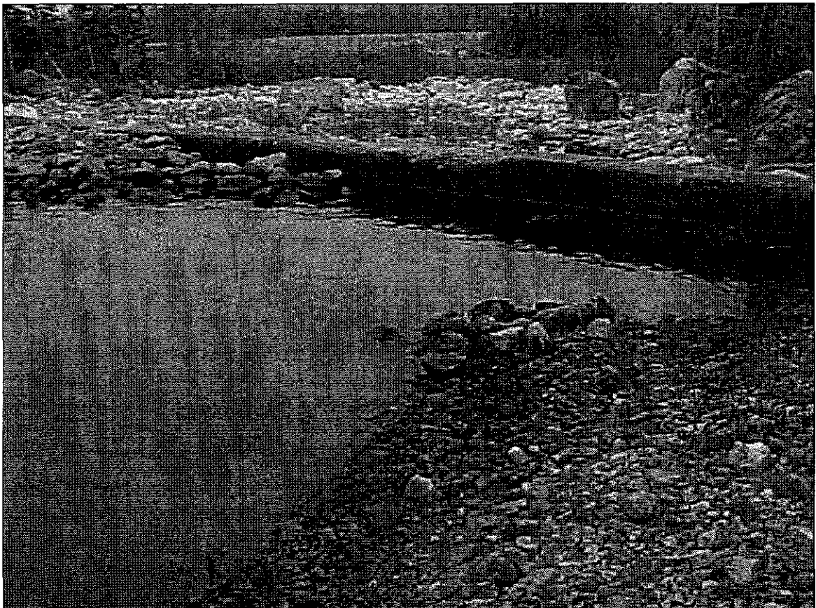
Seal cove Forebay Spillway – Crest With Missing Rock Fill
