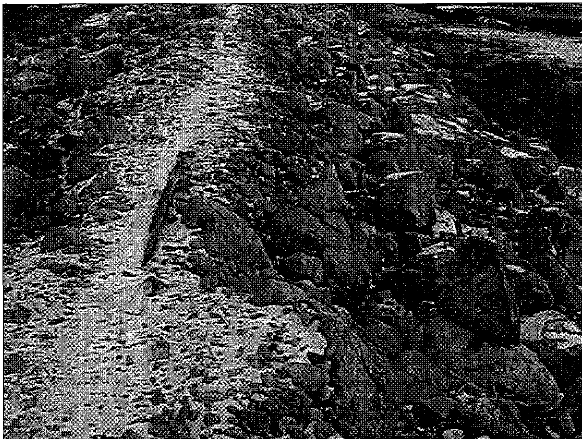
Erosion at Fenelons Pond Dam Crest
